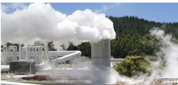
Deep drilling delivers the power
